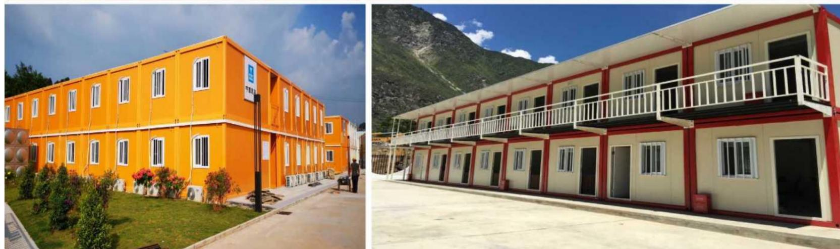
This product is customized and modularized with national standard steel. The amount of steel used is not less than that of the steel structure workshop. The color of the skeleton steel can be customized according to the user, such as Snow Mountain White, Zhongjian Blue, Construction Engineering Red, Engineering Gray, etc. Computer color matching, the frame is sprayed after pickling and phosphating, and the anti-rust and environmental protection grades meet the national standards.
